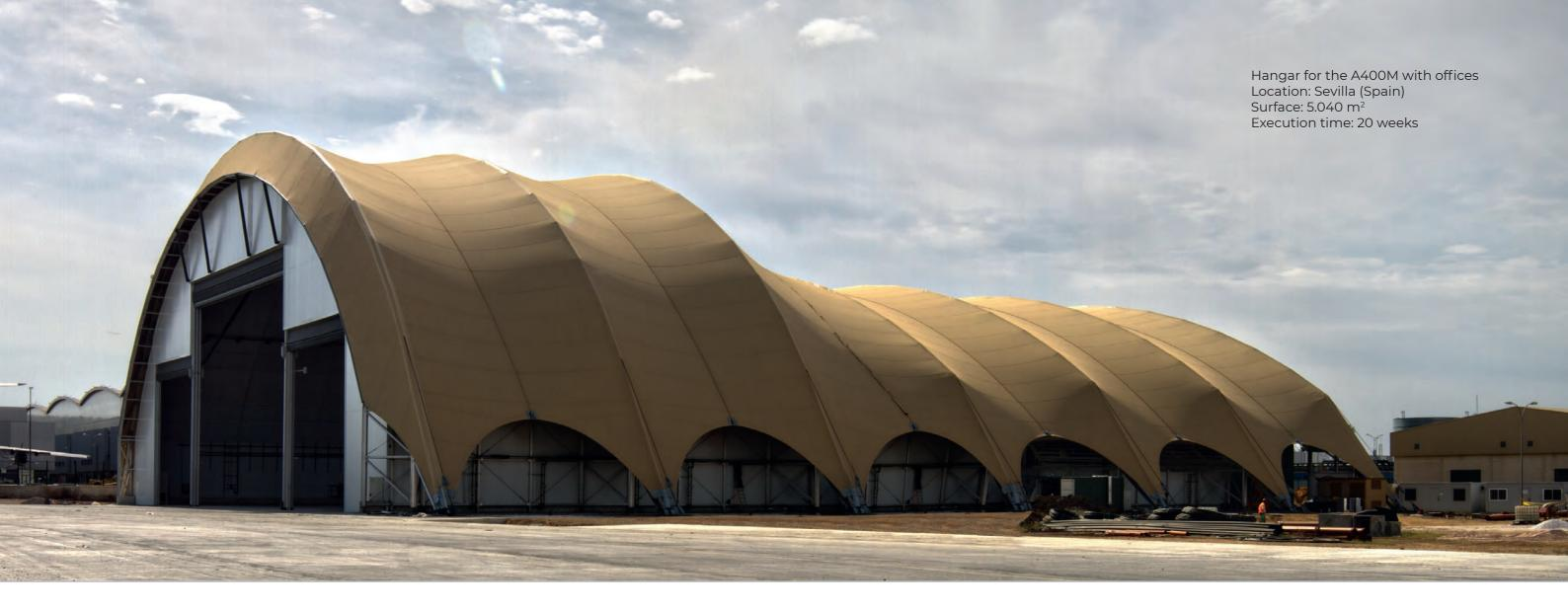
The structures are composed of structural aluminium profiles with mechanical joints.
